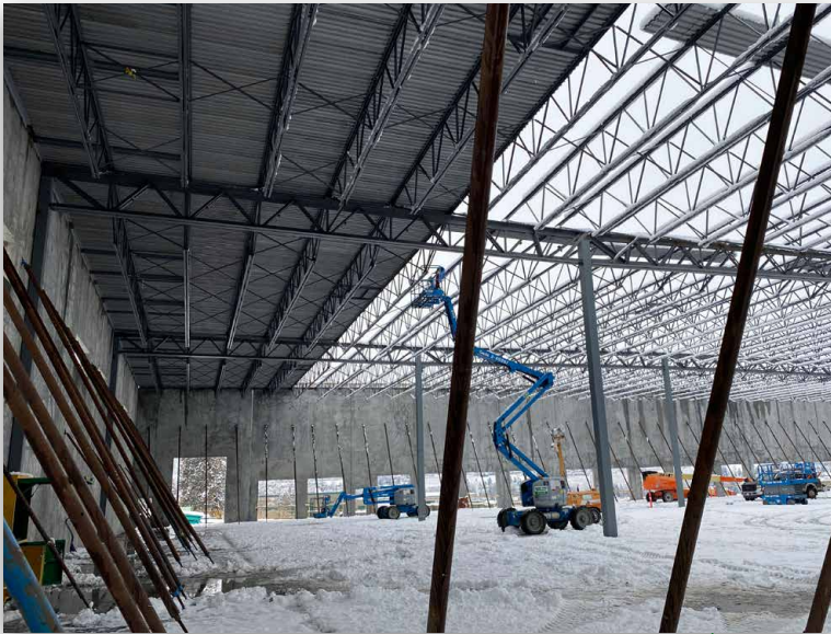
STRUCTURAL STEEL & TRUSS Installation
